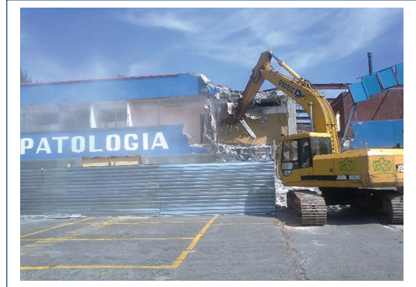
Figure 3. The Pathology Service, as the building it had occupied for many years, was demolished.
