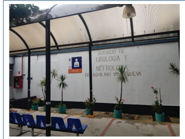
Figure 1. External wall of the Urology Service 105-A.
